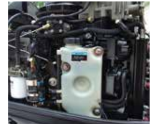
Outboard marine engines shield electrical wiring from high heat engine exhaust.
