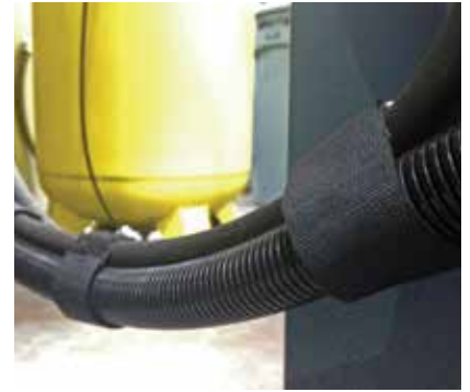
Vibratory hoses in manufacturing environments use Grip Straps to bundle expensive electrical lines.
