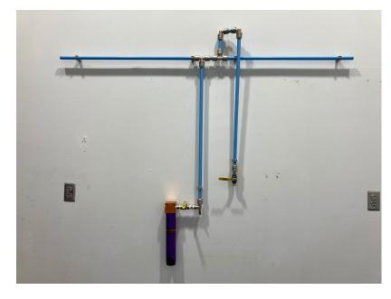
The Tsunami Water Separator can be mounted in-line or with a mounting bracket, directly off the drip leg.
